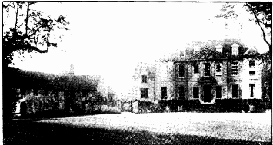
Tickencote Manor 1947. Guest house on left. Still in use.
